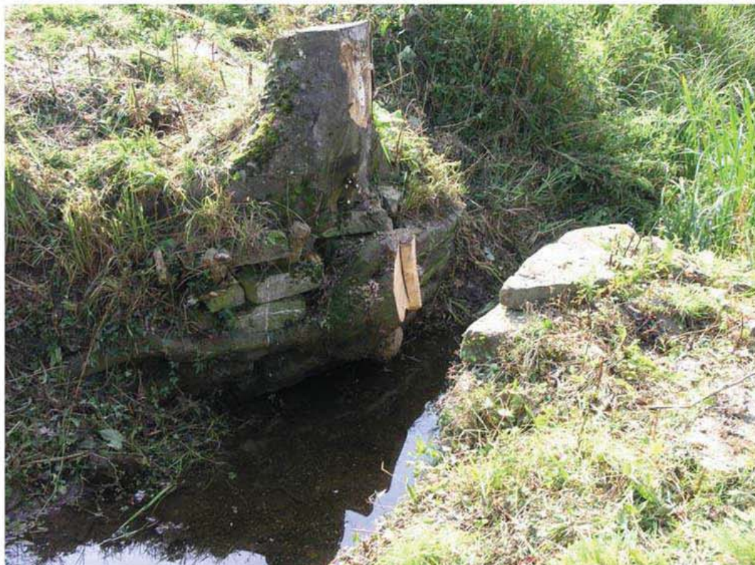
Figure 1: Sluice structure from southeast, i.e. upstream (after Hoverd et al , 2005)
