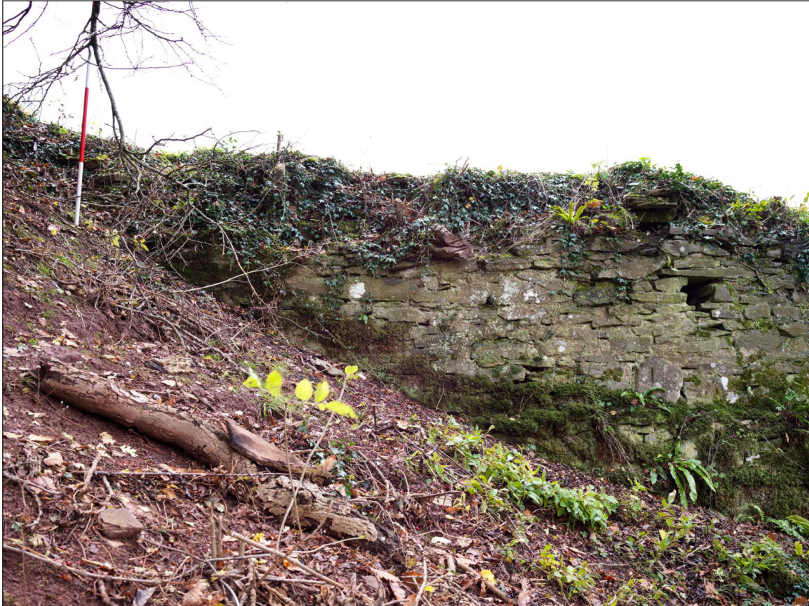
Figure 21 North wing wall, view from south (DP195360).
