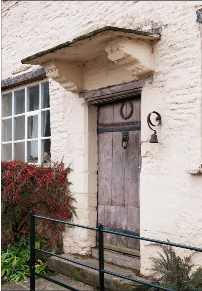
Figure 26 Snodhill Court, doorway to north elevation (DP195444).
