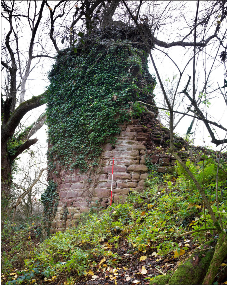
Figure 24 North Tower, view from west (DP195357).
