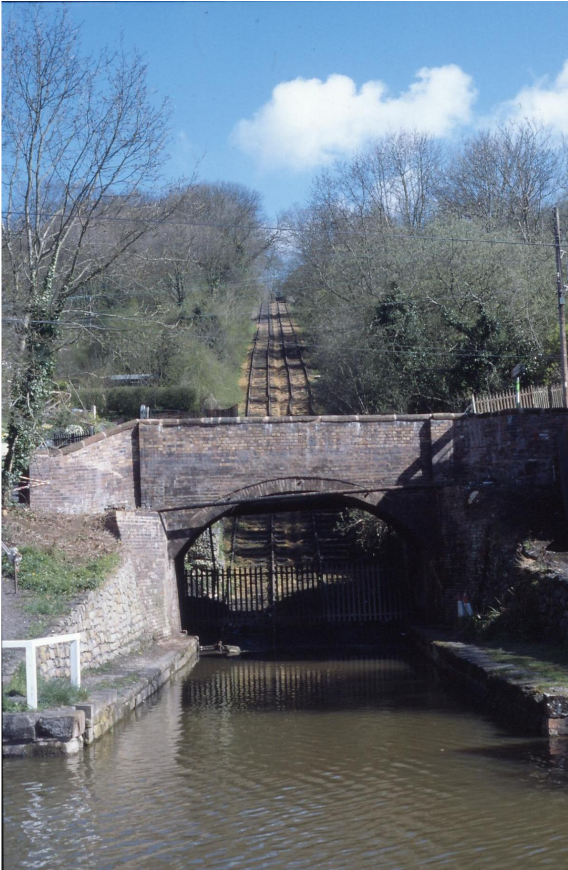
Railway and canal technology influenced each other considerably from the 1790s onwards; the Hay incline in the Severn Gorge is a railed incline connecting two stretches of canal.
